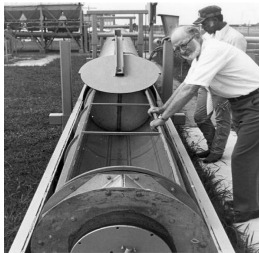
Figure 1: Dr M.R. Carstens with a 40 inch prototype for Tubexpress at the Georgia Institute of Technology[6].
